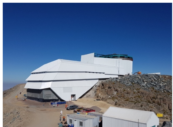
Figure 1.1 LSST in construction on Cerro Pachón in February 2018 (Credit: LSST)
